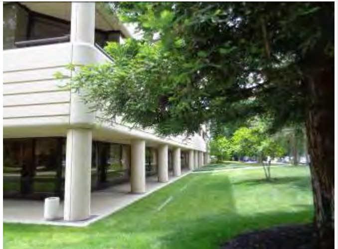
10. View of south and east sides of Building 2440 – facing north
