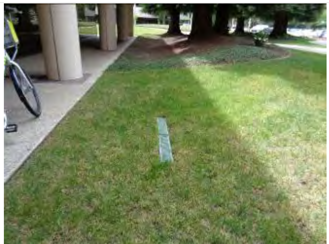
18. View of stormwater drain in landscaping
