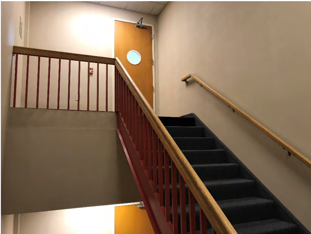
Photograph 16: Example of staircase in the Property building.
