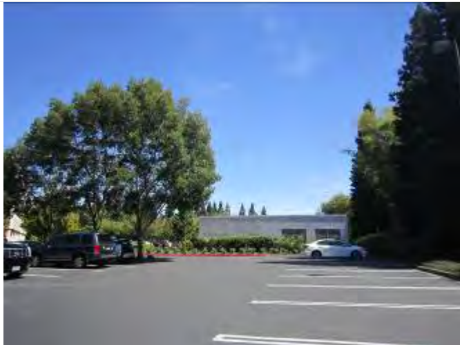
15. View of back-up generator housing – facing south
