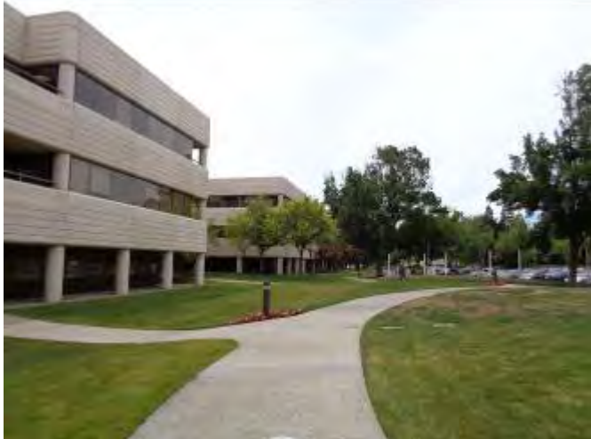
7. View of west side of Buildings 2430 and 2440 – facing south
