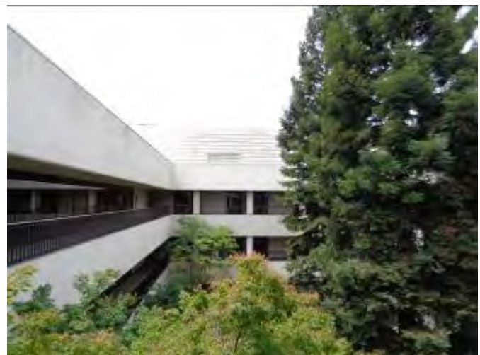
6. View of second floor level of Building 2420
