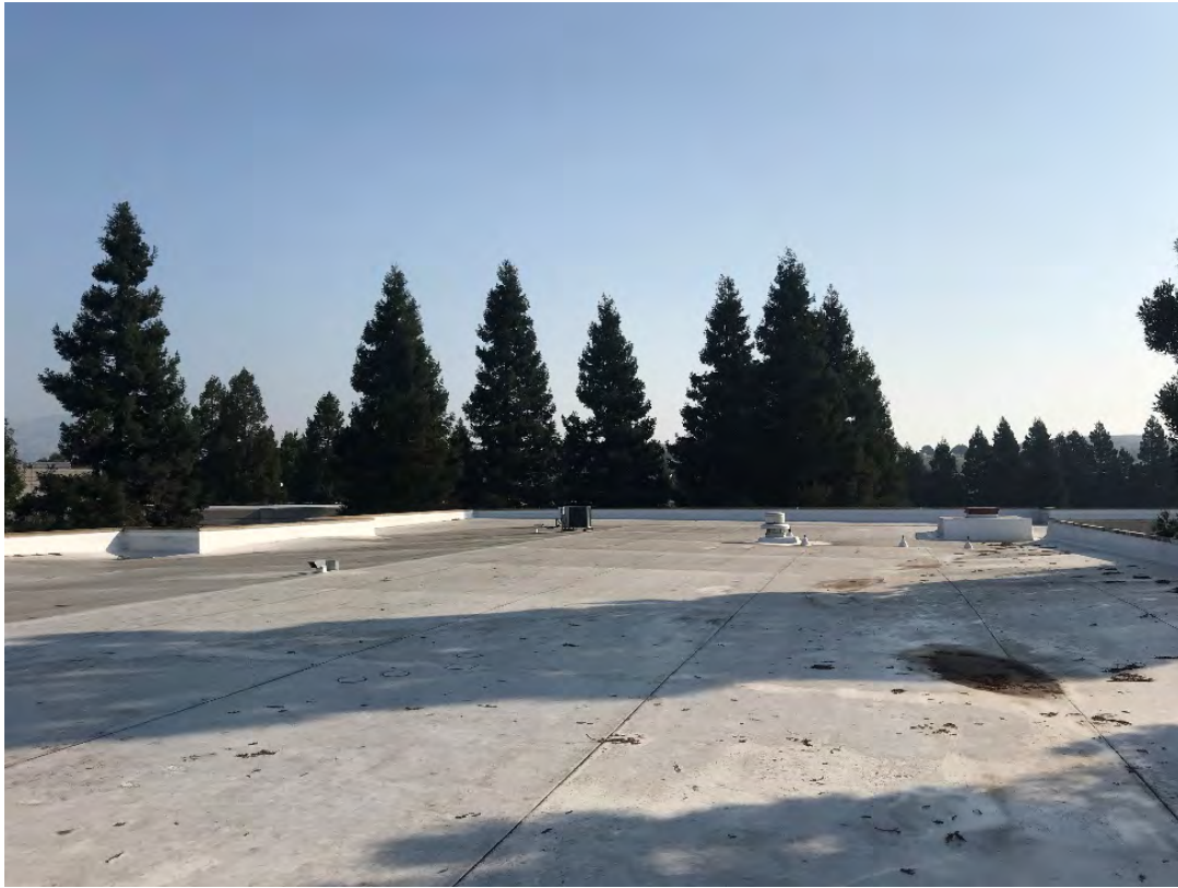
Photograph 27: View looking east from the roof of the Property.
