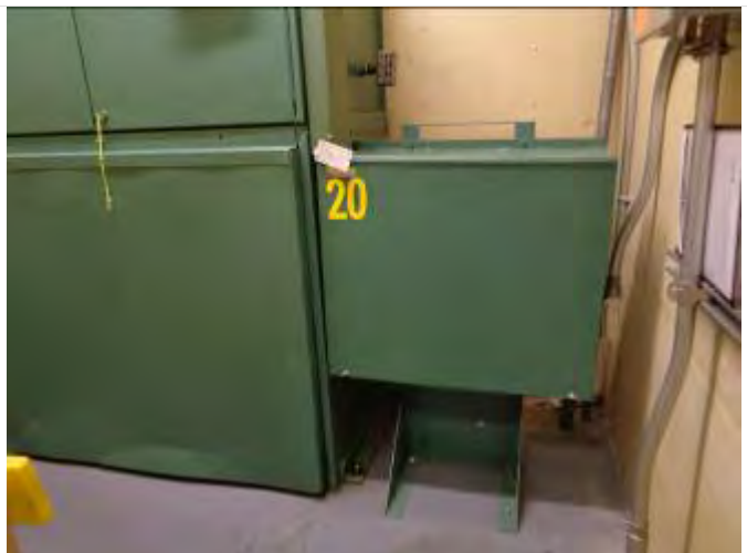
42. View of elevator equipment for Building 2440
