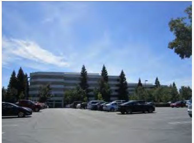
48. Adjacent site to the west – facing west
