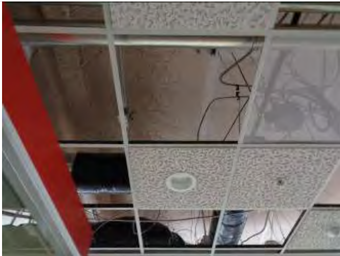
21. View of vacant Suite 390 – Building 2400
