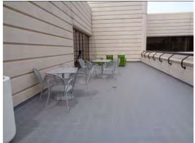
22. View of representative exterior terrace area between Buildings 2400 and 2410
