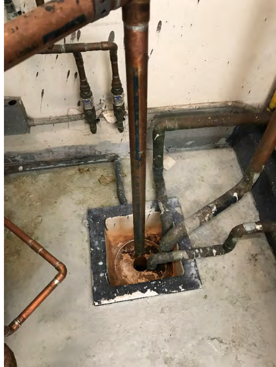
Photograph 32: View of boiler room drainage system located on the roof of the Property.
