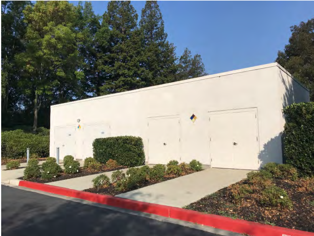
Photograph 7: Exterior of the backup diesel generator building.
