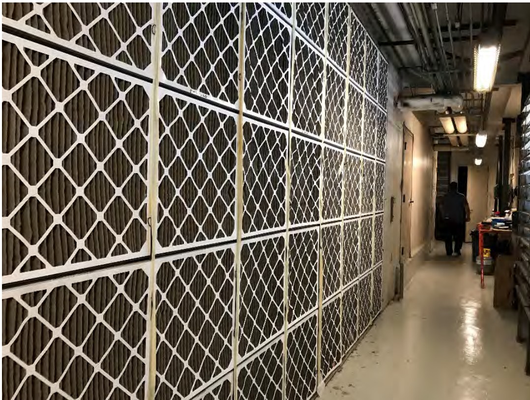
Photograph 28: View of HVAC filtration system located on the roof of the Property.
