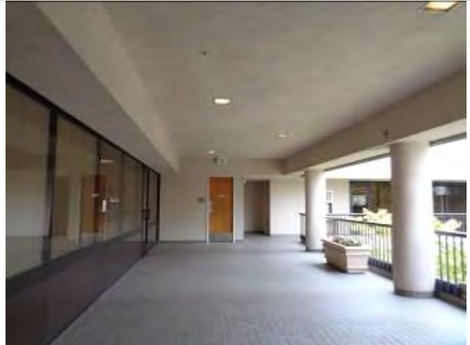
32. View of second level walkway – Building 2420
