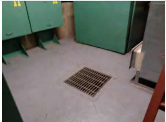
28. View of floor drain in elevator equipment room
