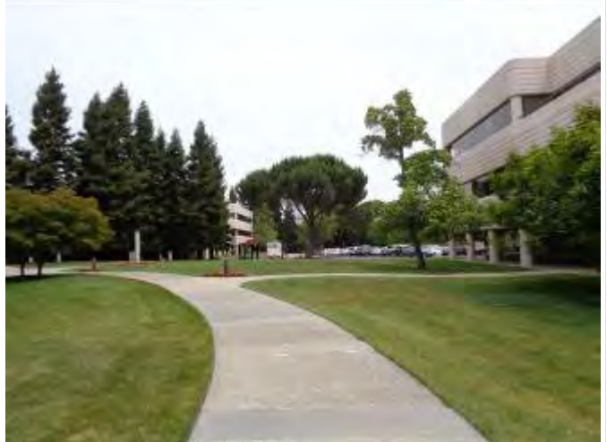
8. View of south side of Building 2420 – facing north
